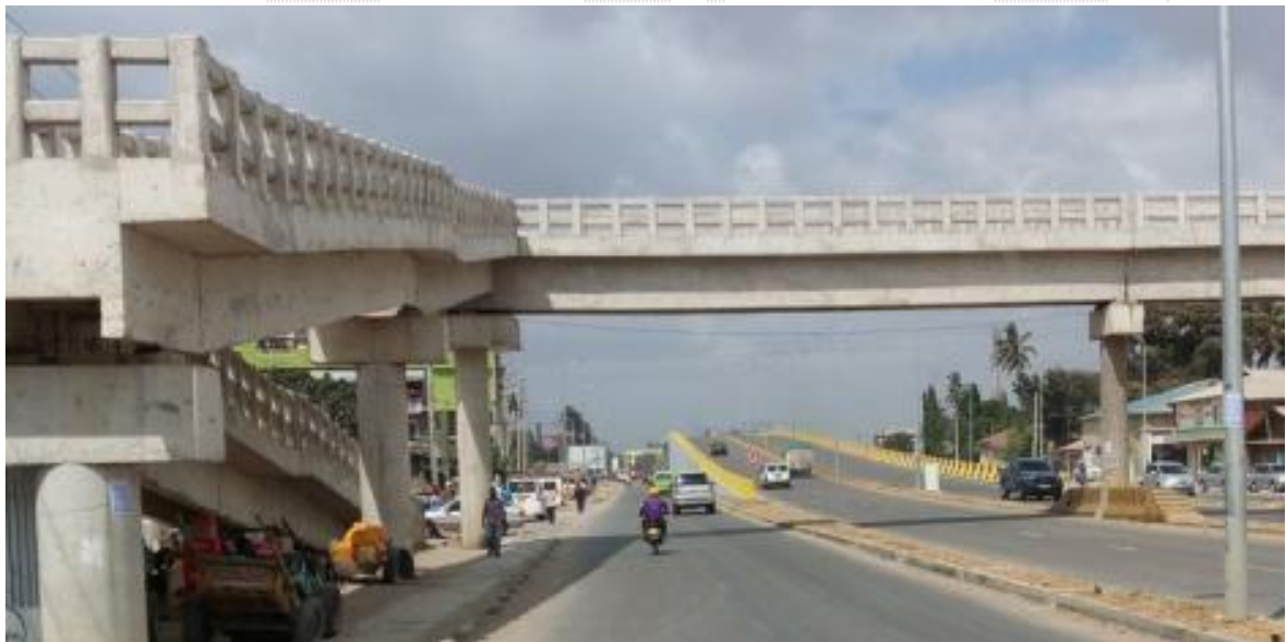
Figure 26 newly constructed Port Reitz road section
