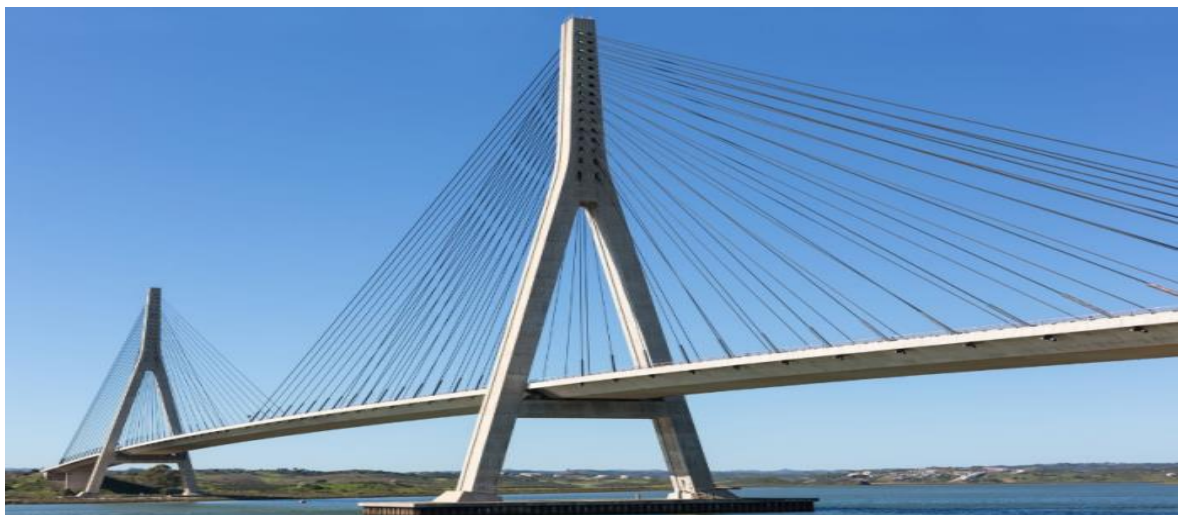
Figure 28 One of East Africa's most impressive infrastructure the recently opened 525-metre long Source of the Nile Bridge
