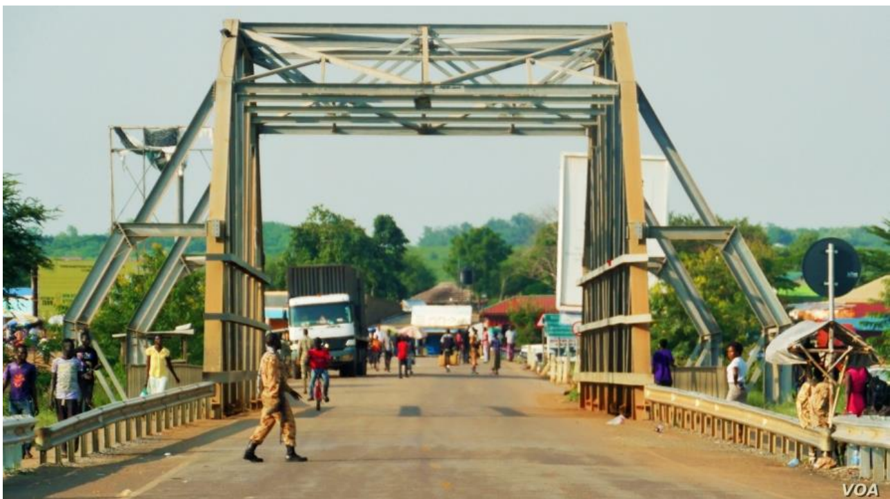
Figure 33 The Nimule Bridge – source VOA
